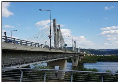
Sejong Haknarae Br. Walkway(Cable Stay Br., Under Conc. Box Girder, 700x9.0m)
