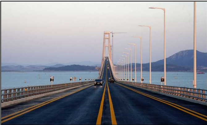
11km Chunsan Grand Br.(Motorway w/o Walkway). Underside Walkway Feasible w/ Composite Deck
