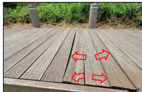
Gap Opening, Bumps on Wooden Decks
