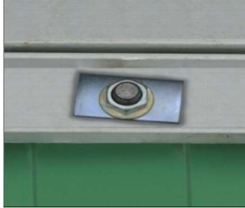
Connecting Deck to Girder with Welded Stud Bolts
