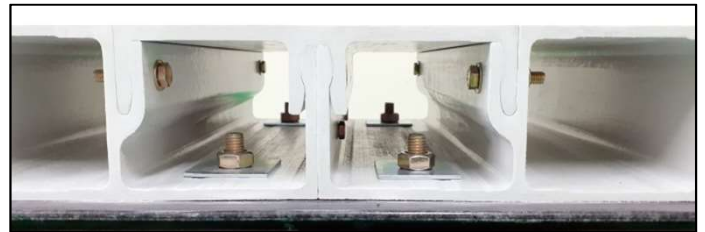
Bolted at Snap-Fit(Prevent Gap-Opening & Disconnections)
