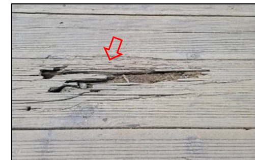
Rot and Segregation of Wooden Deck
