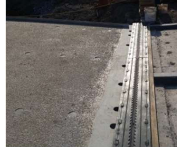
Installing Expansion Joints
