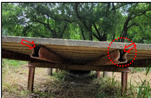
Vulnerable Connection of Wooden Deck
