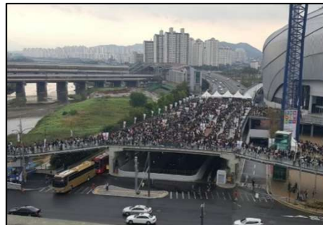
Walkway around Gochuck Skydome Baseball Stadium(Plate Girder Br., 410x7.4m)
