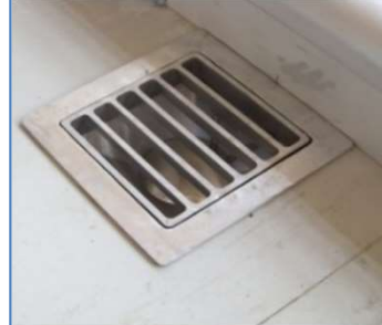
Installing Drainage Pit
