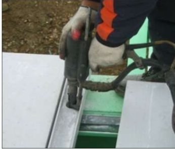
Welding Stud Bolts to the Girder with Stud Gun
